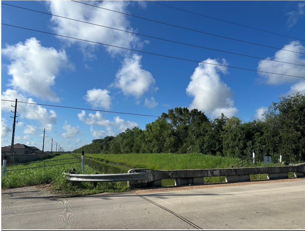
Looking south from Old Massey Ranch Road at the drainage canal.
