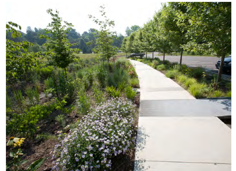
Bio-swales, similar to drainage ditches, utilize selected vegetation to filter and slow down stormwater runoff prior to its drainage into the watershed. These bio-swales can be designed using native vegetation adapted to the area, requiring minimal maintenance.
