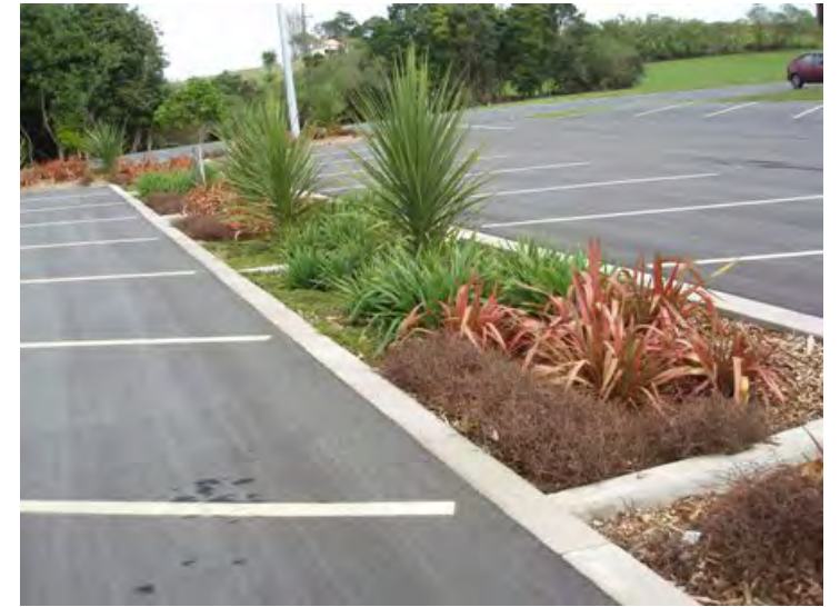
Use of native plants within landscape areas of parking lots can aid in removal of contaminants and sediments from stormwater prior to drainage into the watershed.
