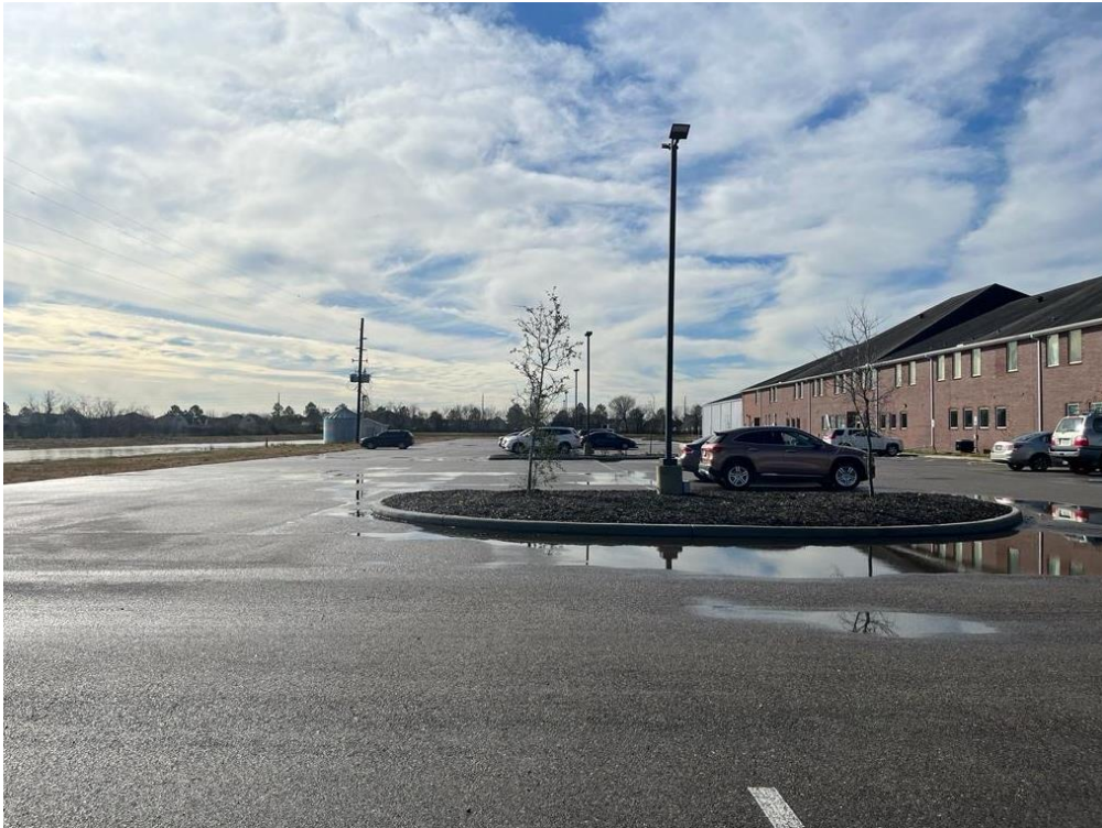
11800 Magnolia – Facing South in main parking lot.
