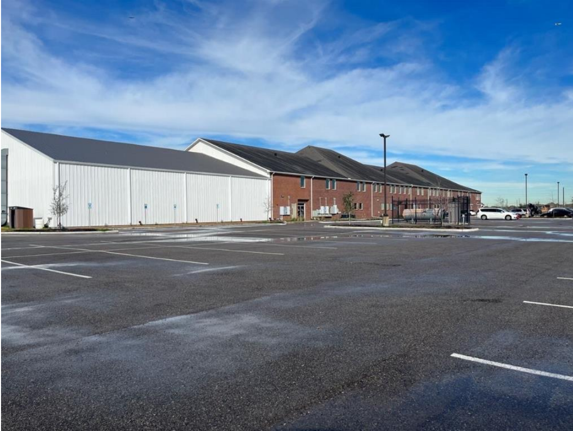
11800 Magnolia – Facing Northwest from main parking lot area.
