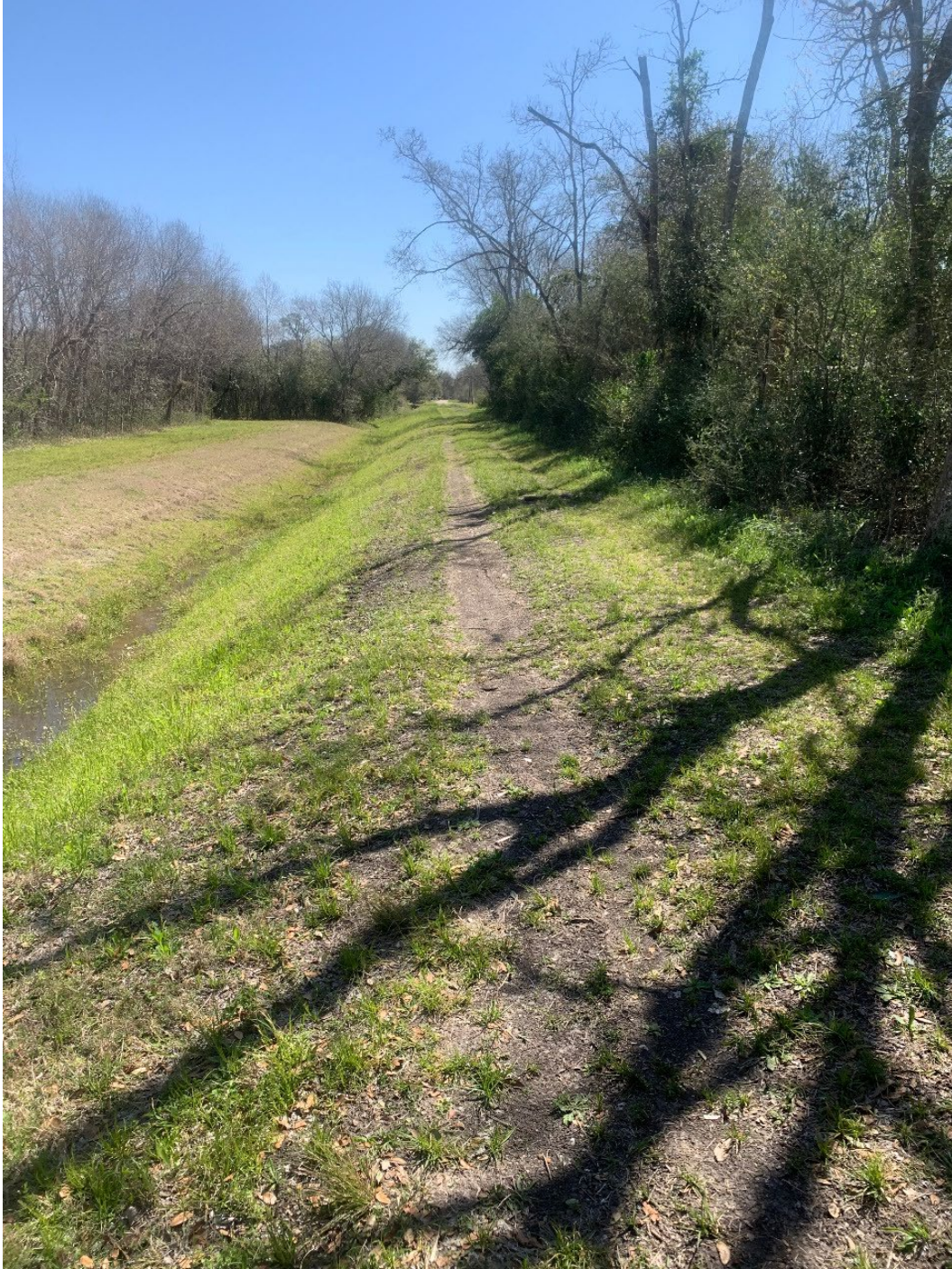
Unimproved Del Bello Boulevard and Drainage ditch
