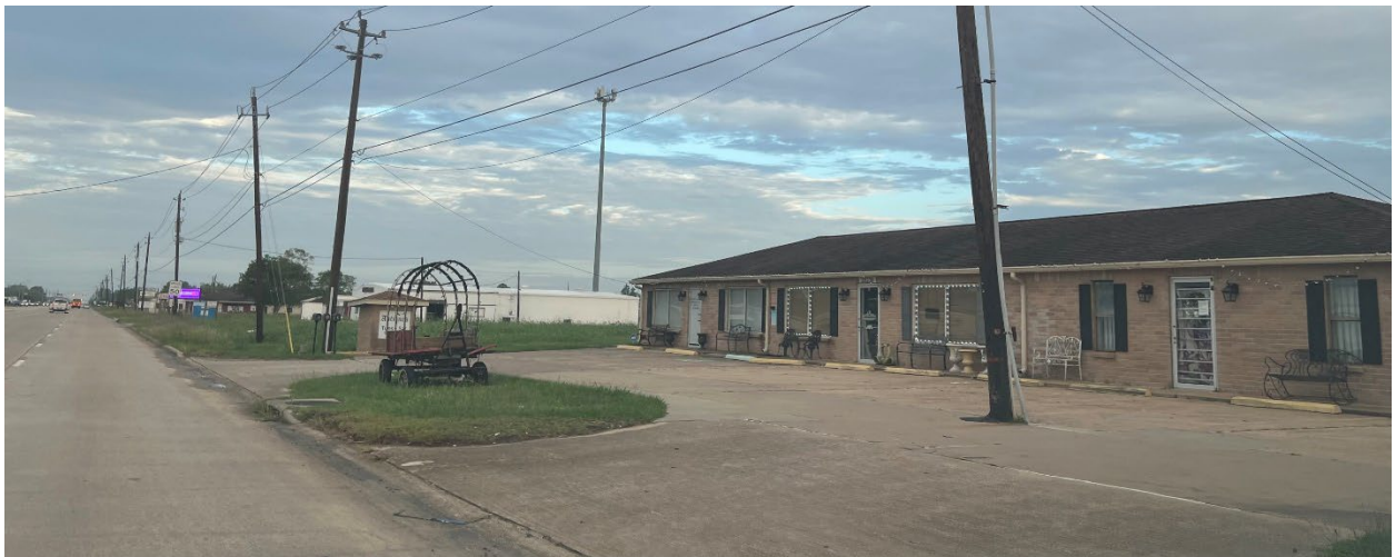
View of commercial development to the north across from Highway 6
