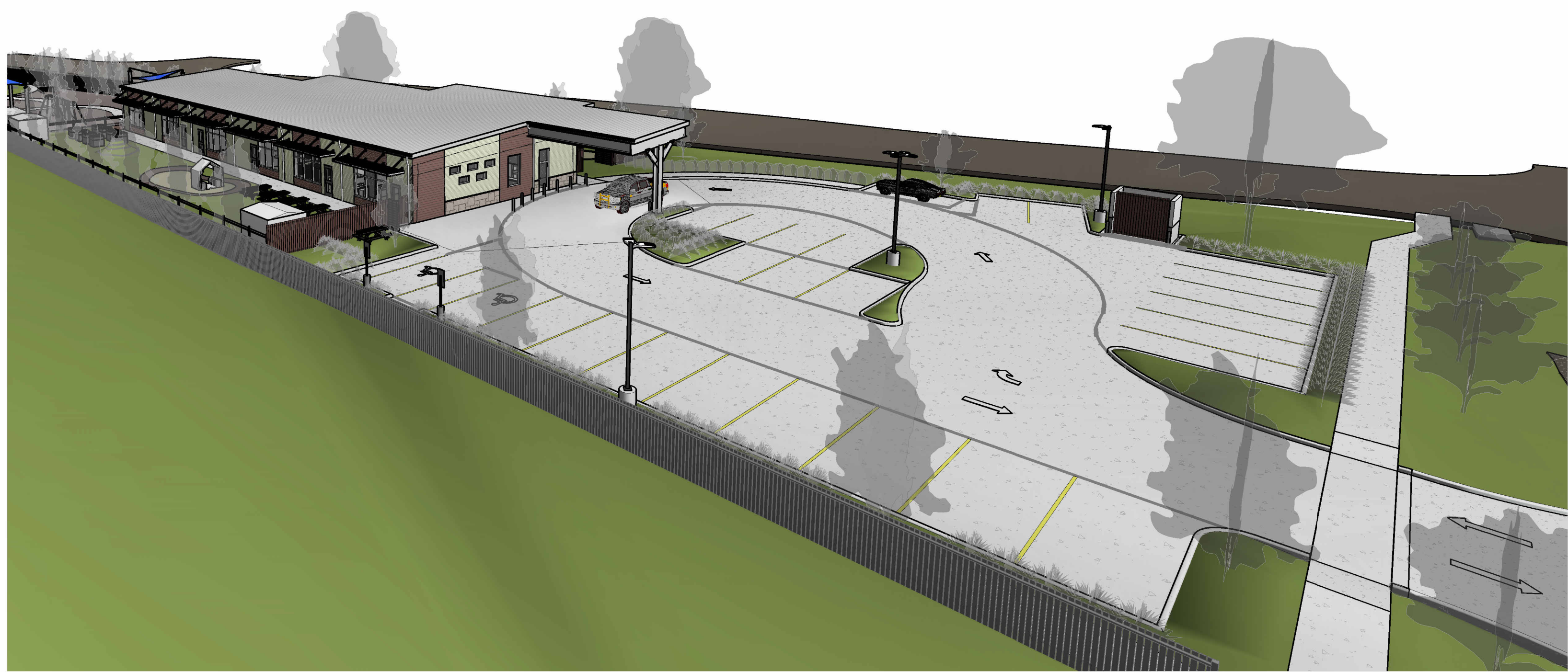
3 AERIAL VIEW FROM SOUTHWEST
