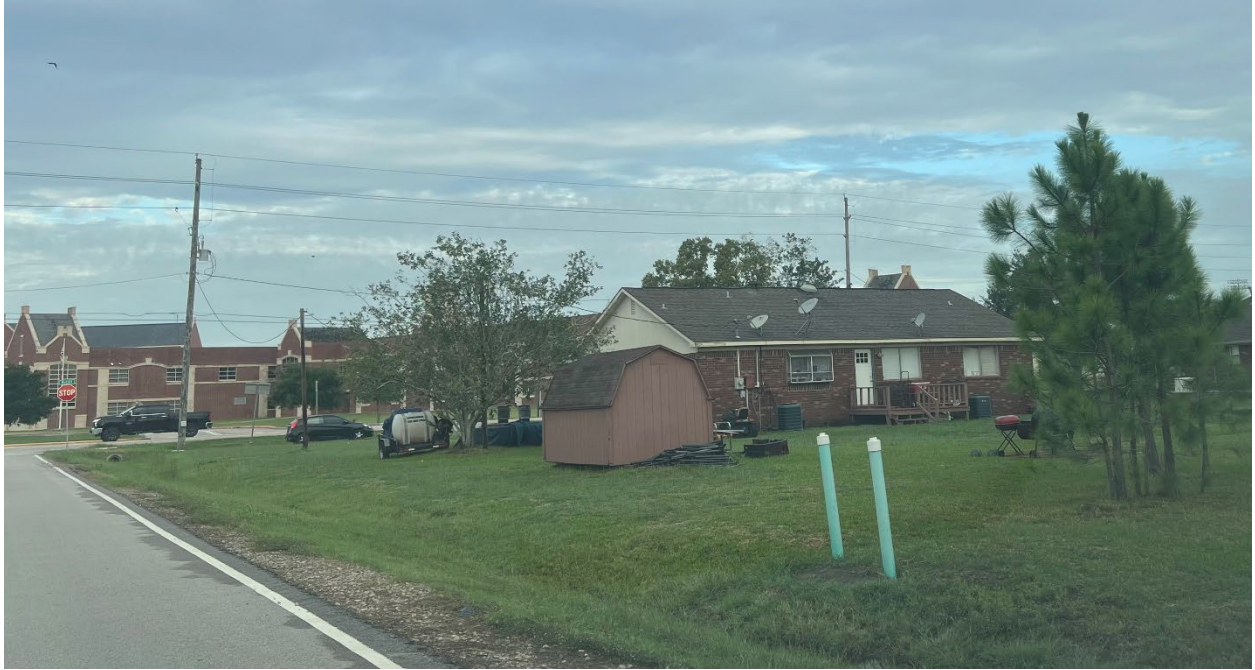
View of the legal nonconforming residential (Light Commercial) property looking from Large Ave to the north-west
