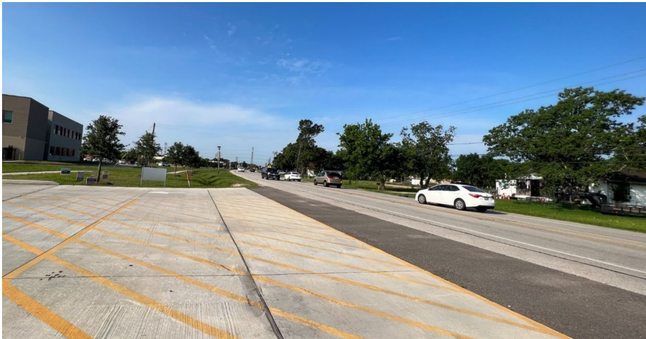
Viewing N Masters Rd from west entrance of E.C. Mason Elementary School to South
