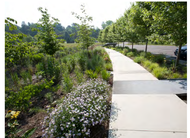
Bio-swales, similar to drainage ditches, utilize selected vegetation to filter and slow down stormwater runoff prior to its drainage into the watershed. These bio-swales can be designed using native vegetation adapted to the area, requiring minimal maintenance.
