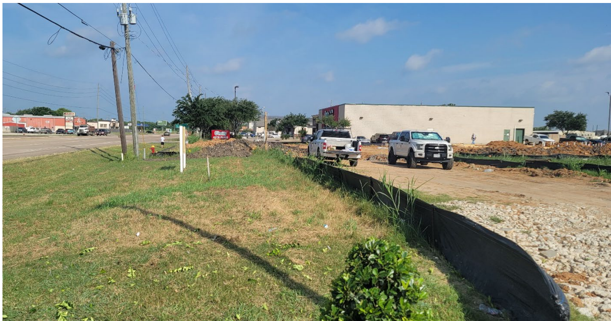
View of the HWY 6 Right-of-way along the subject site and adjoining property
