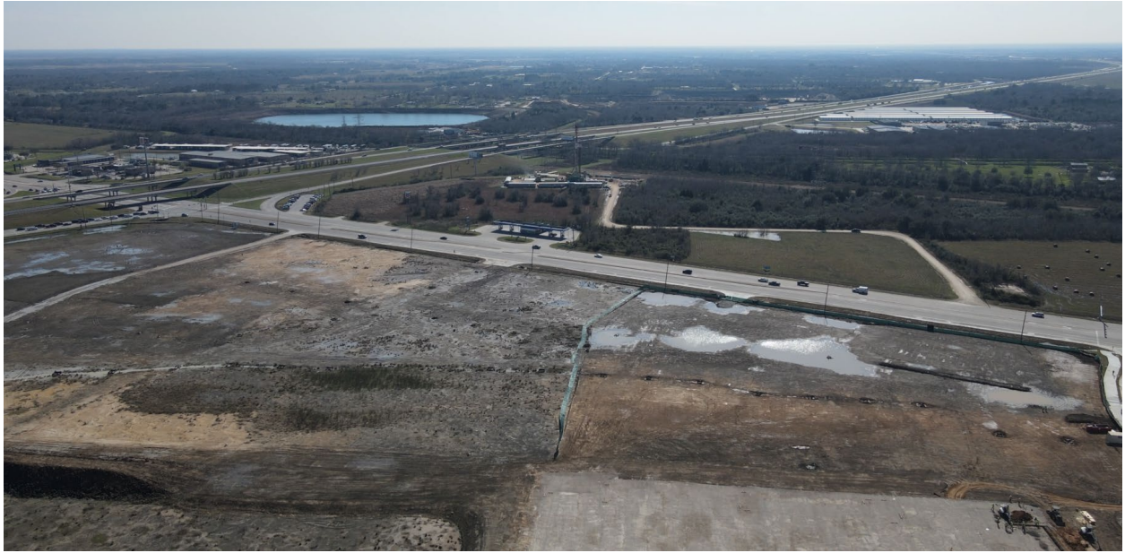
Aerial view (viewing South) of Manvel Town Center Site
