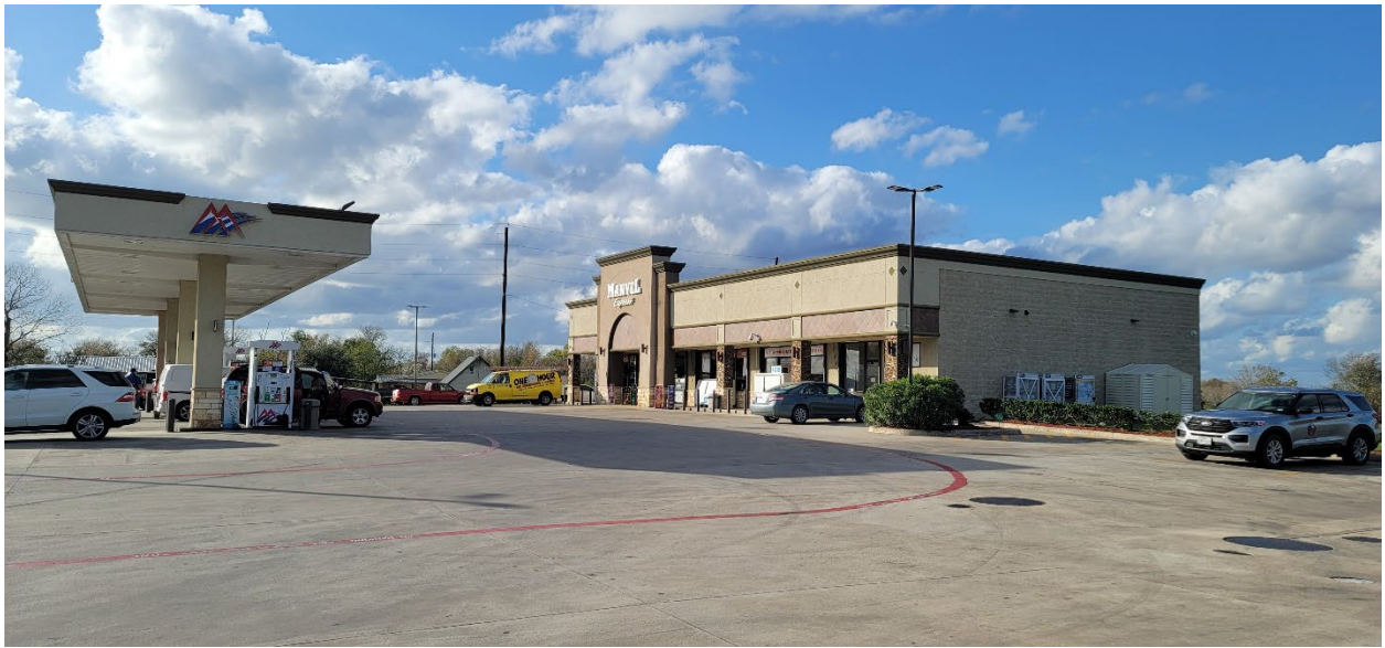
View of the existing Gas station and convenience store from south-eastern corner.
