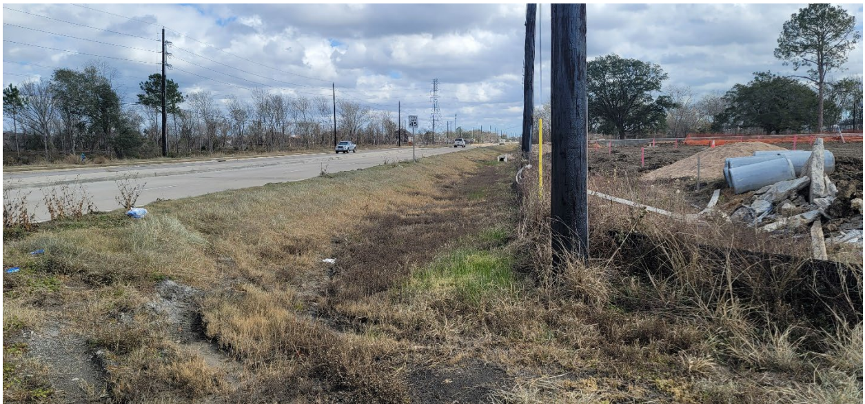
Open drainage ditch along Bailey Rd.
