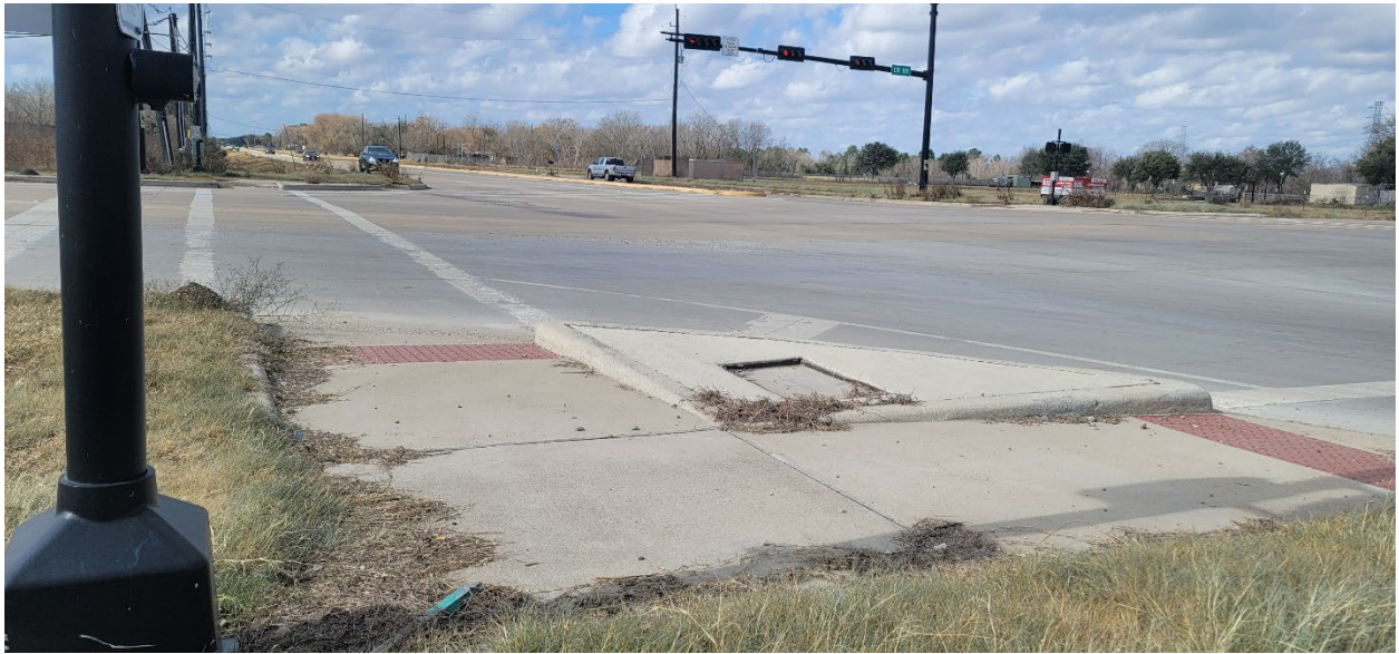
Existing Sidewalk landing pads at intersection abutting subject site
