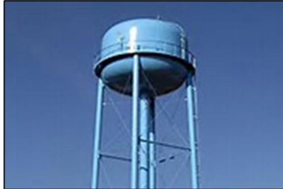
ELEVATED STORAGE TANK
