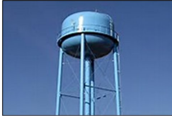
ELEVATED STORAGE TANK
