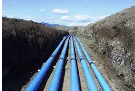
WATER PLANT IMPROVEMENTS
