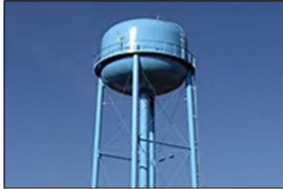
ELEVATED STORAGE TANK
