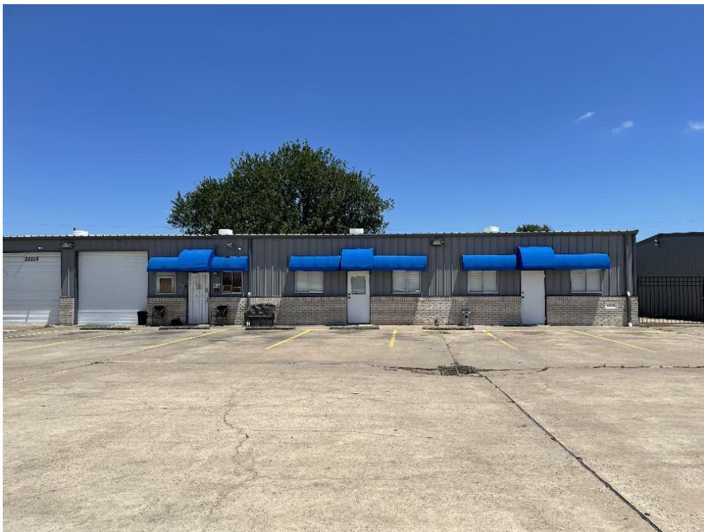
Subject property from SH 6 (existing building with closed game room).
