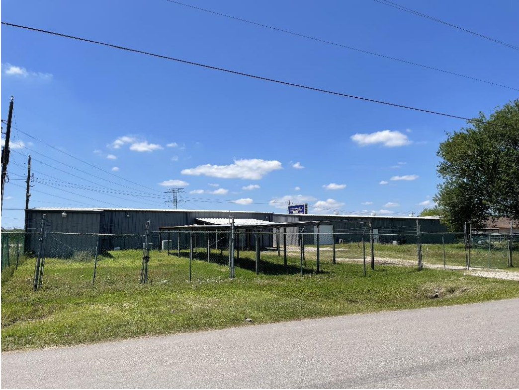
The rear of subject property from Mustang Bayou Road.
