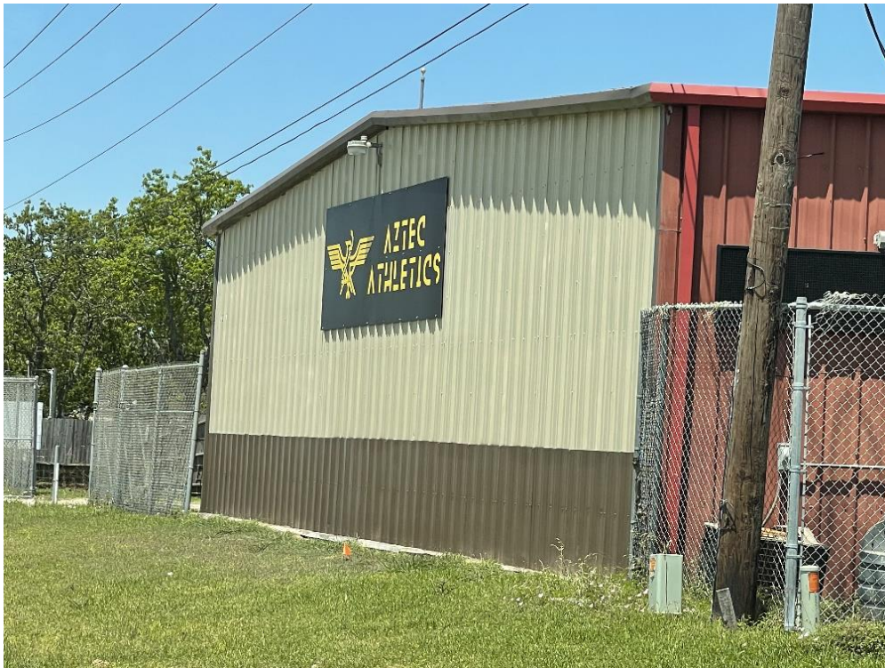
Abutting commercial property to the west (along SH6).
