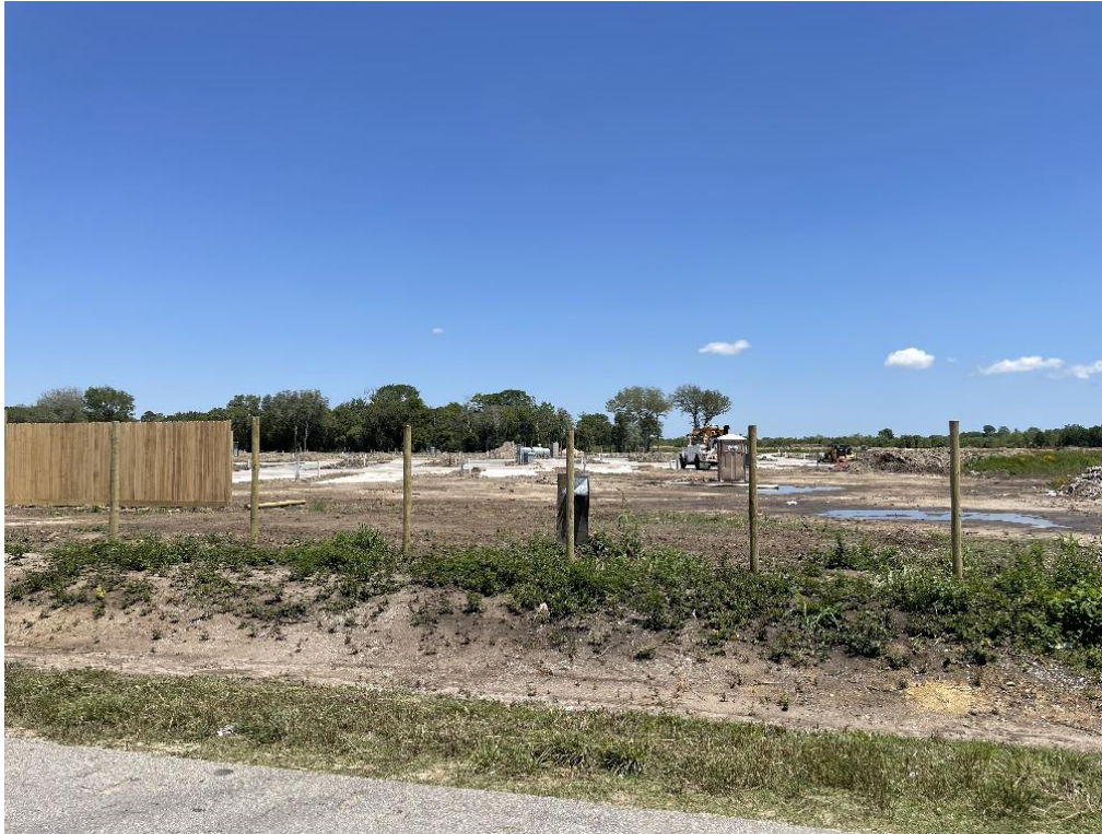
RV Park under construction on the north side of Mustang Bayou Road.
