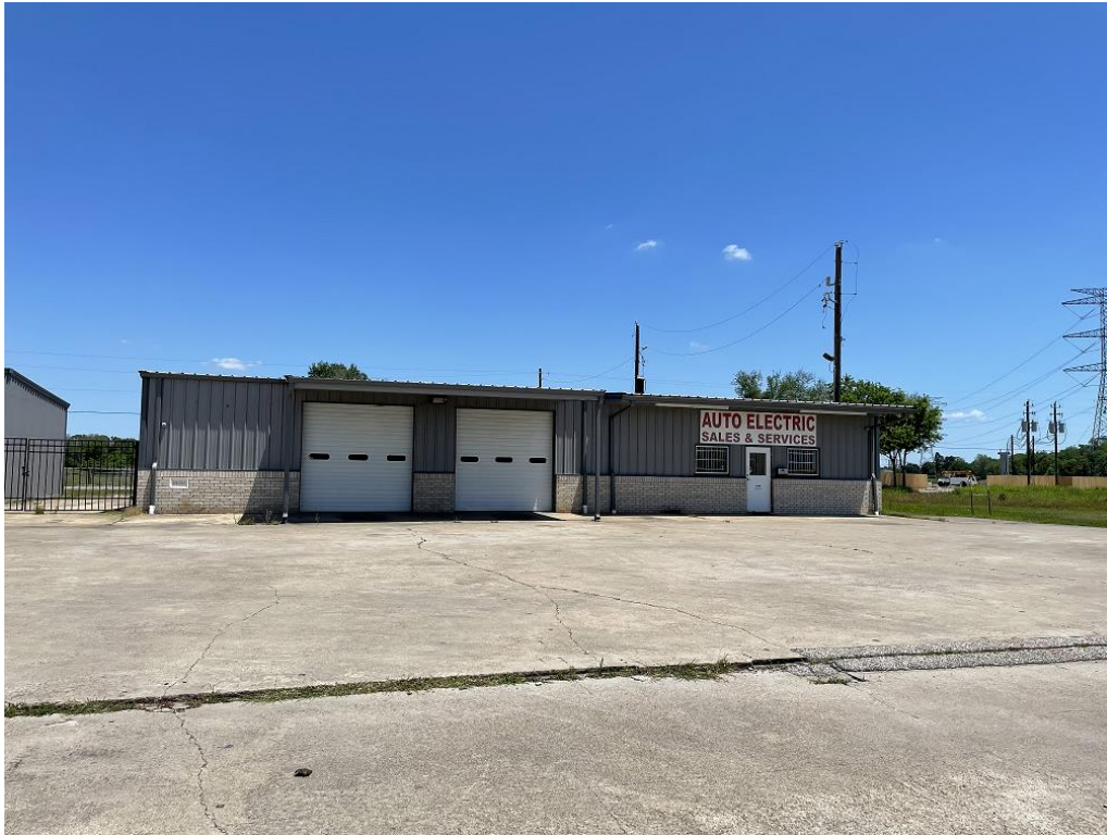
Subject property from SH 6 (existing building with automotive repair).
