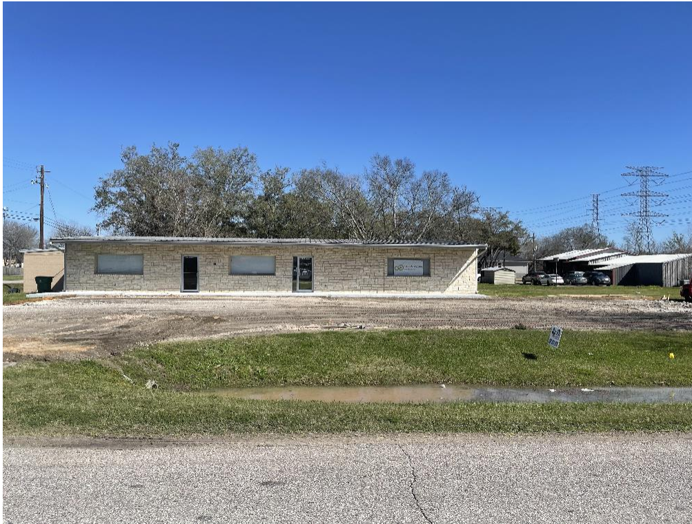
Looking at abutting property from Masters Road (east) at the current parking lot construction.
