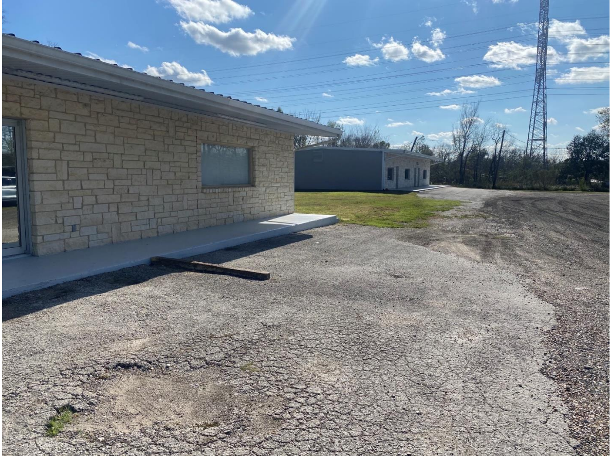
Exhibit 9 Unpaved frontage of Subject Property
