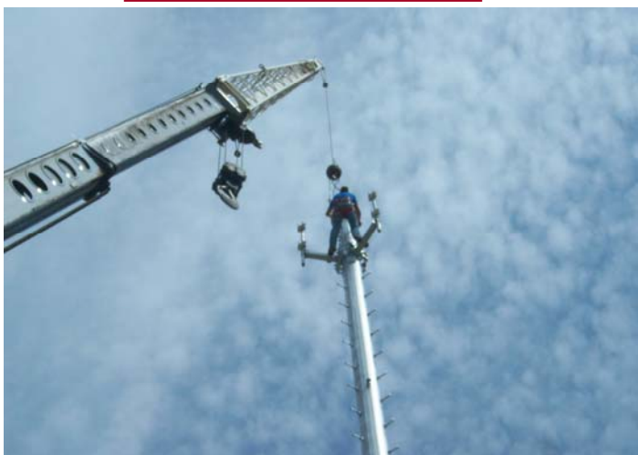
Installation of 115' monopole with antennas in Amarillo, TX
