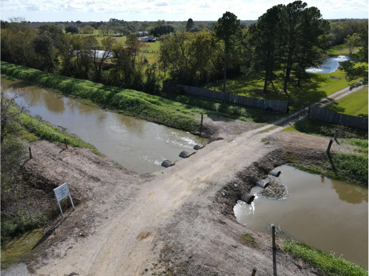
Exhibit 11 Access Easement and Bridge over GCWA Canal to subject property
