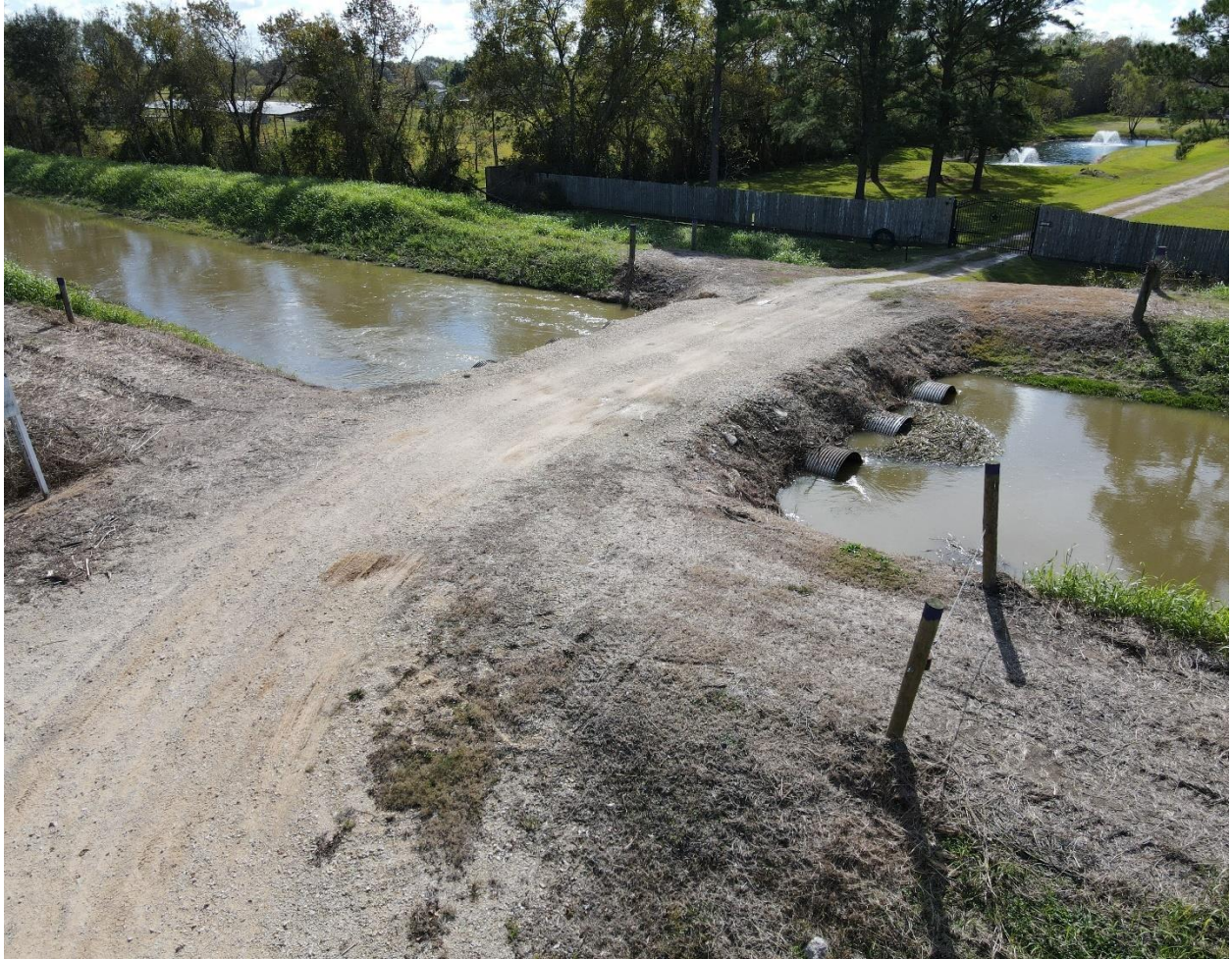
Exhibit 10 Drainage Bridge over GCWA Canal providing access to subject property
