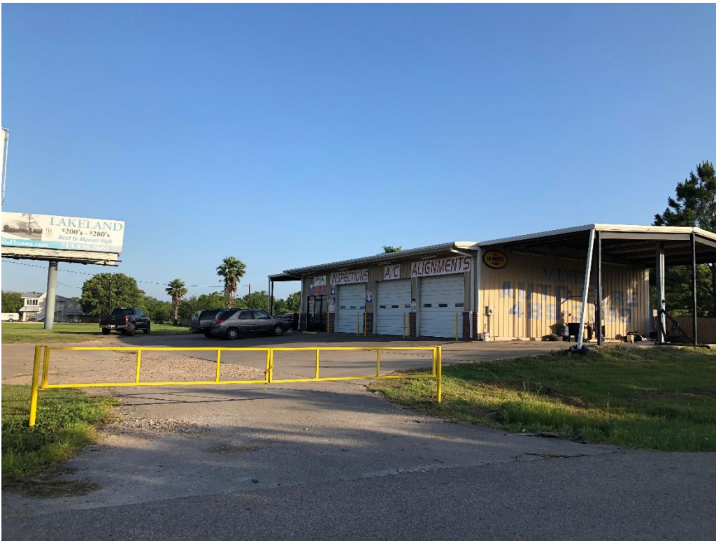
Commercial business abutting the site on SH 6.
