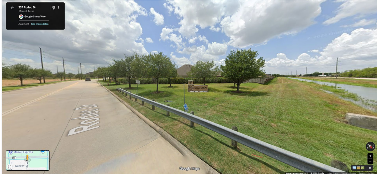
View of the property to the west, across Rodeo Dr (Single Family Residential / Rodeo Palms)
