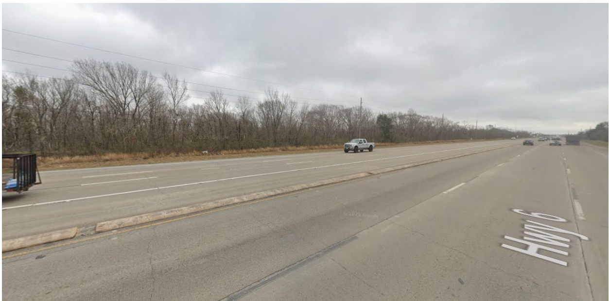
View of the subject site from Highway 6 (south west corner)
