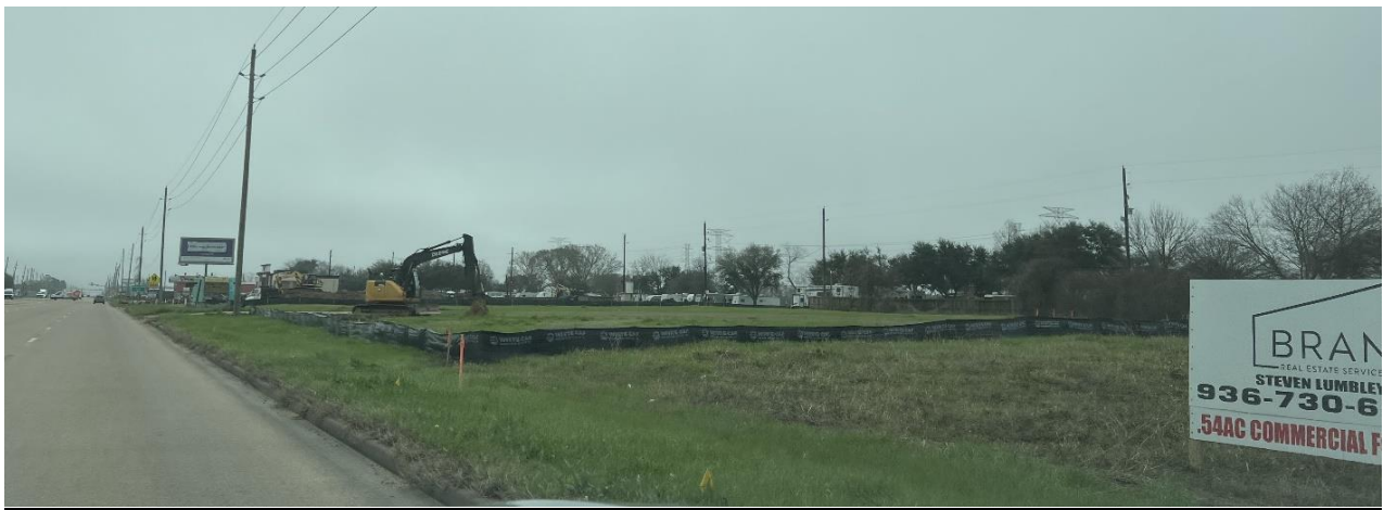
View of adjacent property to the south from Morris Avenue/SH6 (Carwash)
