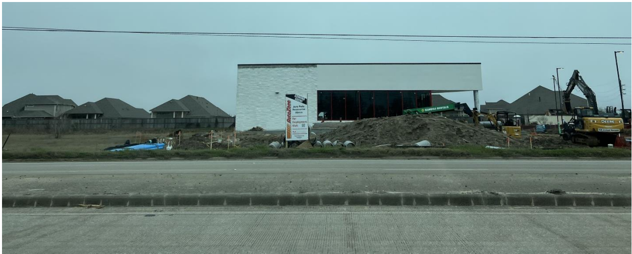
View of adjacent property to the east, AutoZone currently under construction.
